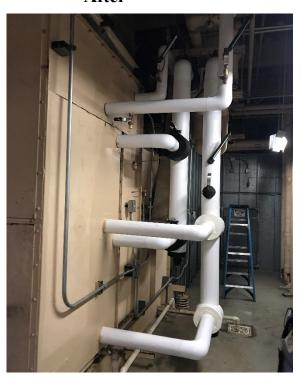
Newly replaced coils and refurbished drain pans on air handling unit
