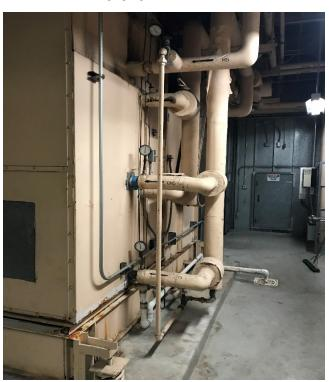
Old failing coils on air handling unit
