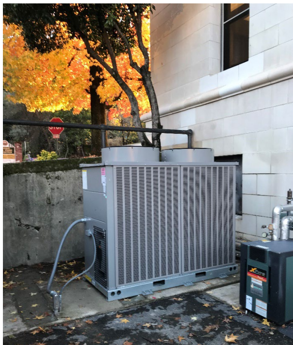
Above: Failing 30-ton chiller unit at Placerville Main Street Courthouse Below: Newly replaced breaker and feeder, and R-410A refrigerant unit
