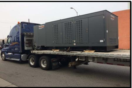
**Before**: Removal of the old generator. The unit weighed over 21,000 lbs., approximately twice as much as the new generator (*above left*).
