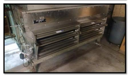
**Before:** Aged air handling unit original to the building's construction in 1958 (*top*).
