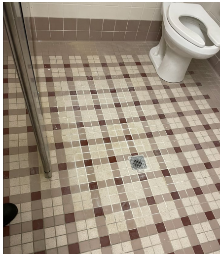
Newly repaired floor drain
