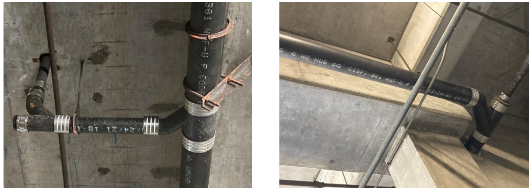
Newly replaced drain pipes and drain lines
