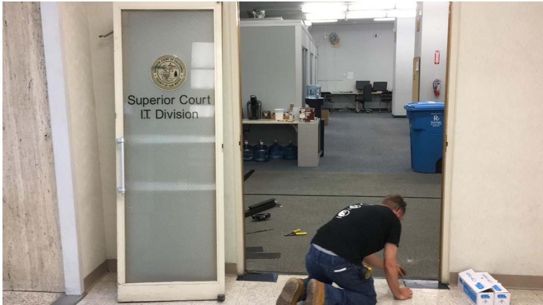
**Above:** Existing doors with wrong swing and no panic hardware are being removed.
