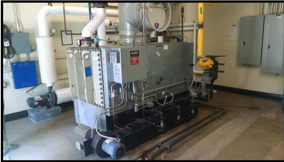
**Above:** Failing existing 3 MBTU Boiler (Parts no longer being fabricated).
