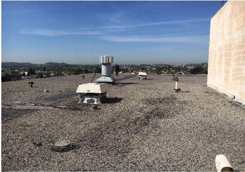
Above: Old roof of Alhambra Courthouse
