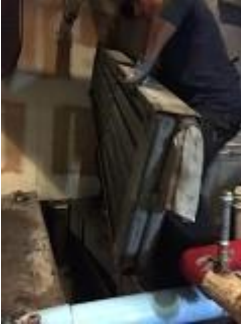
Above: Existing, failing coil Below: Newly replaced coil
