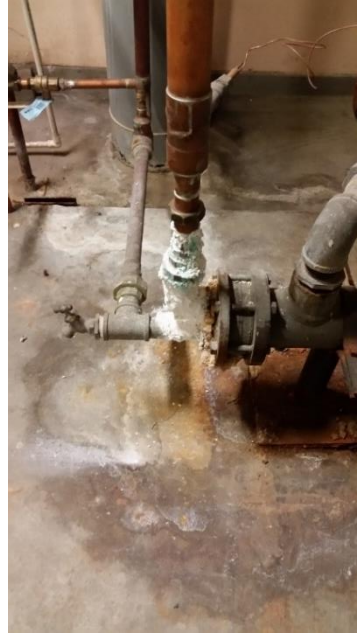
Above: Existing, failing valves and pump Below: Newly replaced valves and pump
