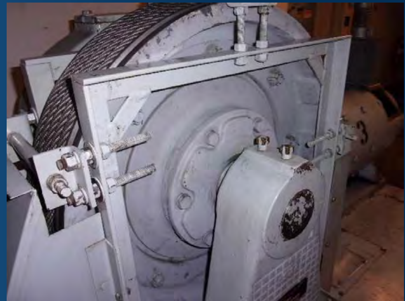
AFTER: Newly sealed hoist motor.
