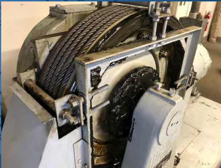
BEFORE: Old hoist motor seal leaking grease.
