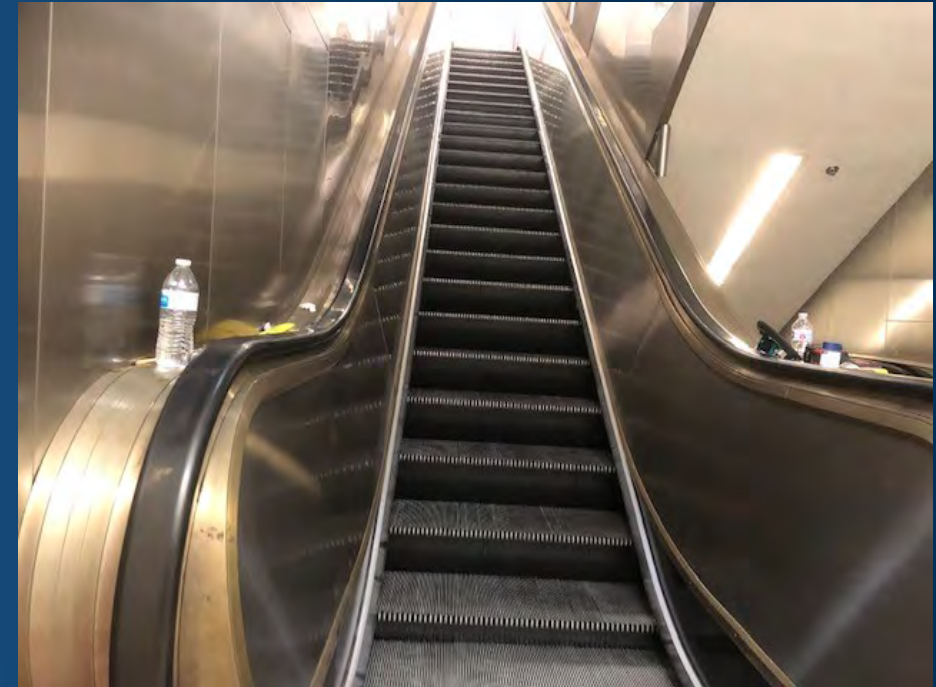
AFTER: Escalator after modernization
