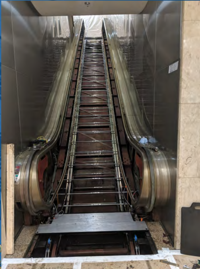
DURING: Escalator during modernization
