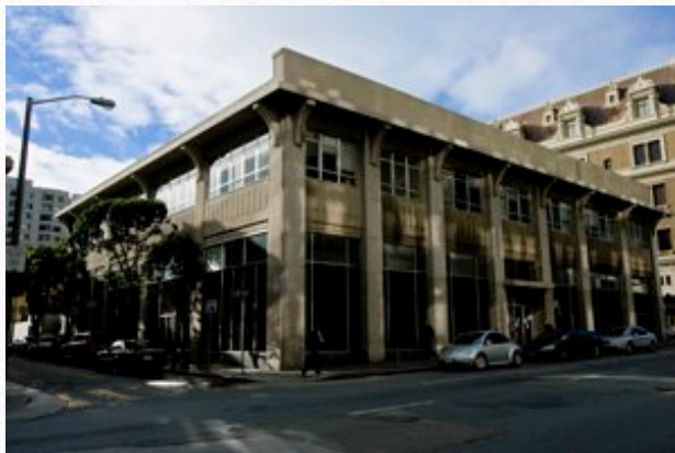
Polk Street Annex
