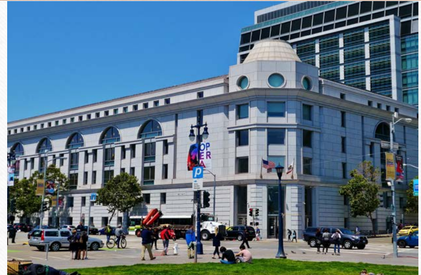
Civic Center Courthouse
